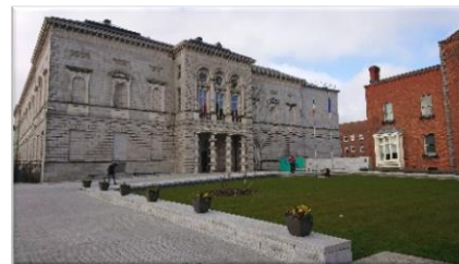
Merrion Square Entrance
